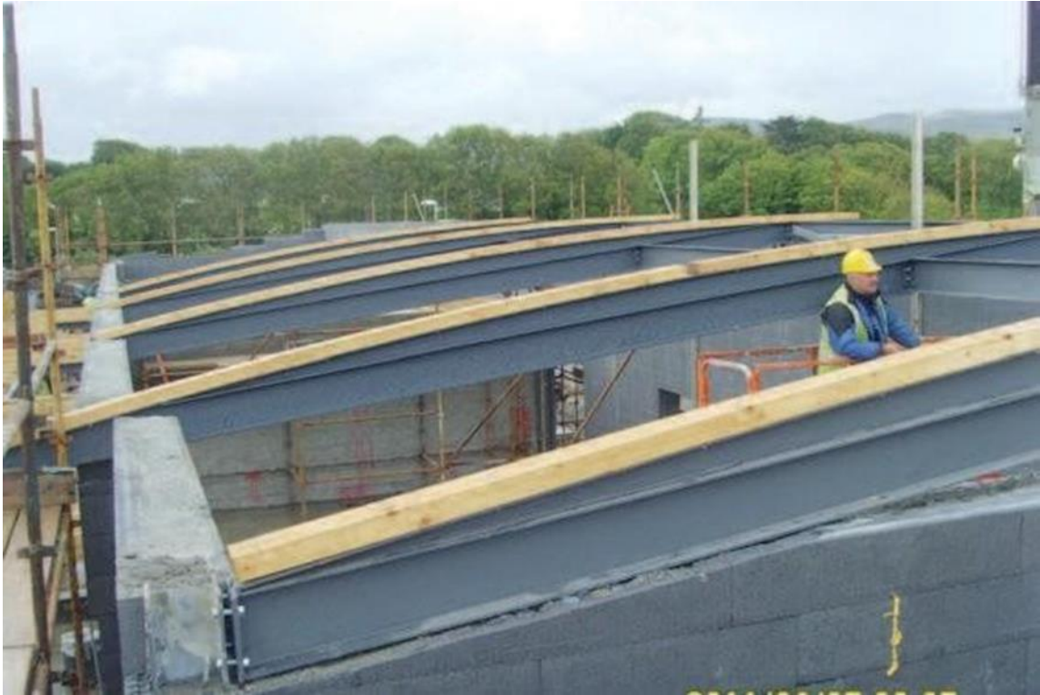
Commercial Building – Showing Previous Structural Column Encased in Wall photo
