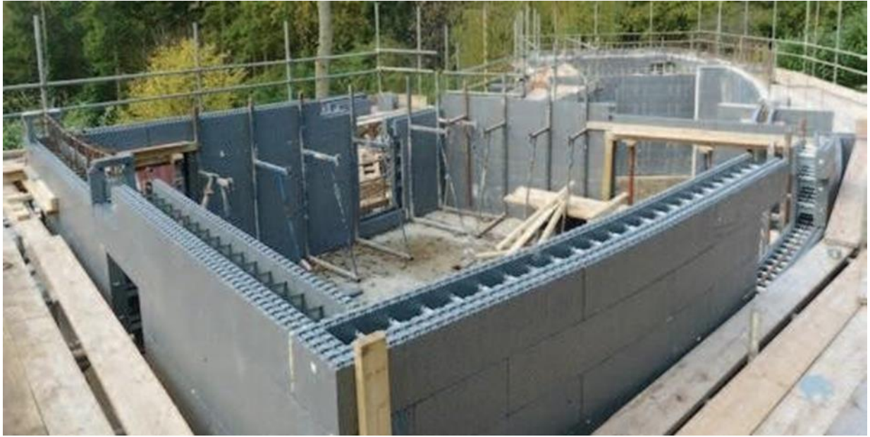
External Curved Wall Construction Photo
