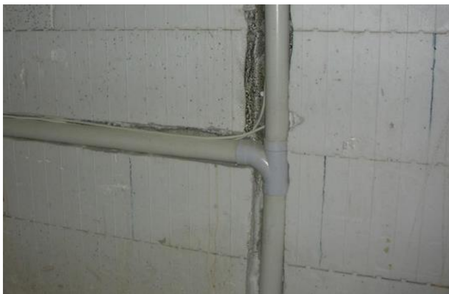
Recessed Pipe or Conduit (max 40mm)
