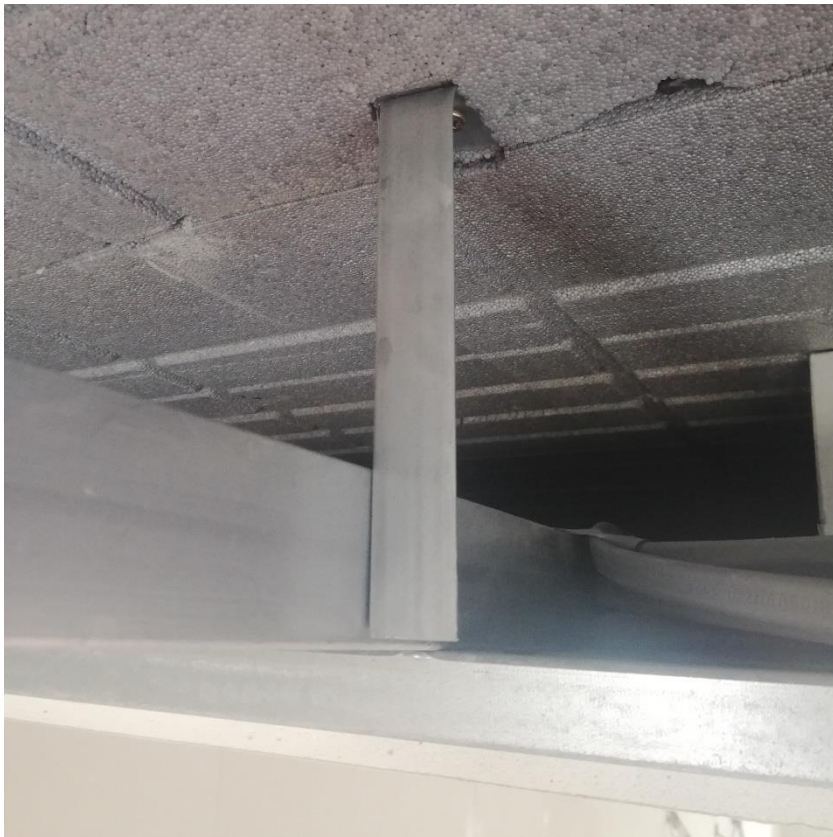
Hanger fixing & typical service void in suspended ceiling.
