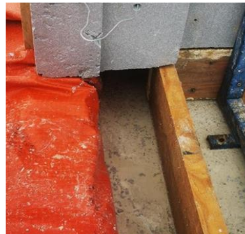
Temporary Wall Shutter at door threshold
