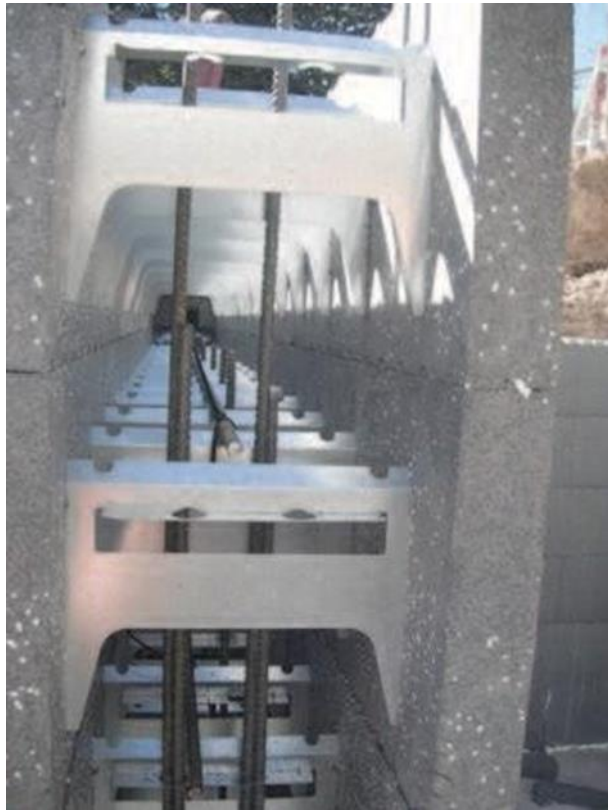
Steel Reinforcement in forms
