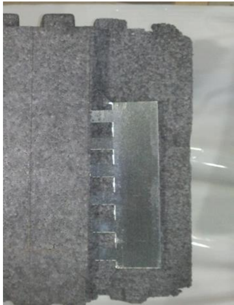
Fixing flange exposed through block
