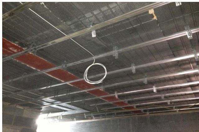
Suspended ceiling showing service void
