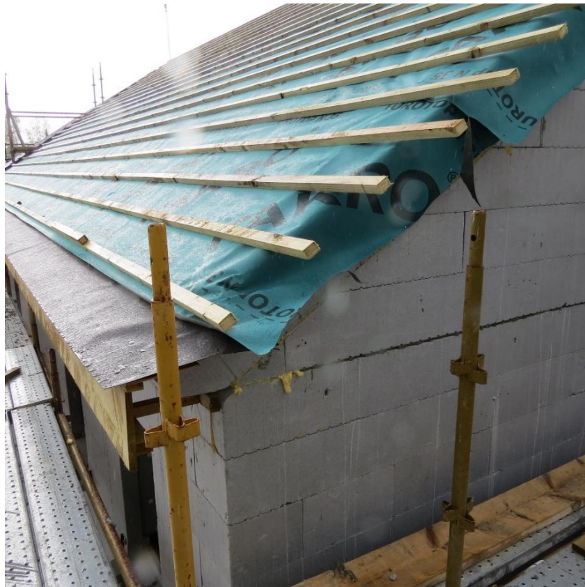
Breathable membrane & Slating/Tiling Batton
