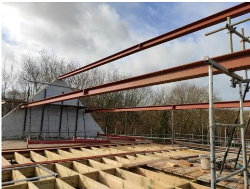
Traditional Timber Joist
