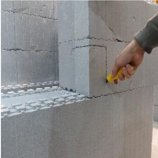
Cutting & removal of plug after marking
