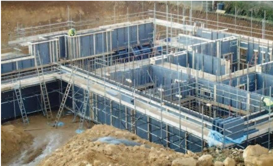
Construction of two storey basement
