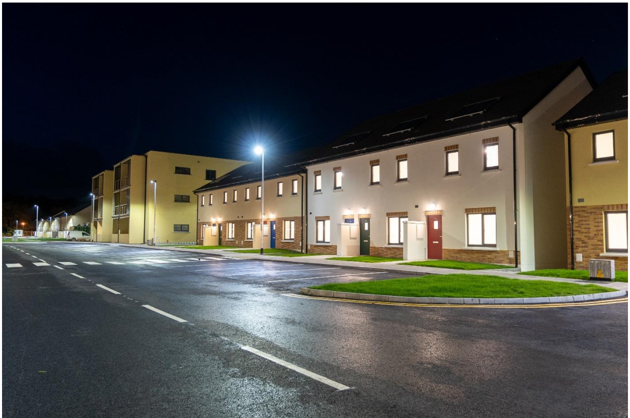
Thermohouse development in Killarney
