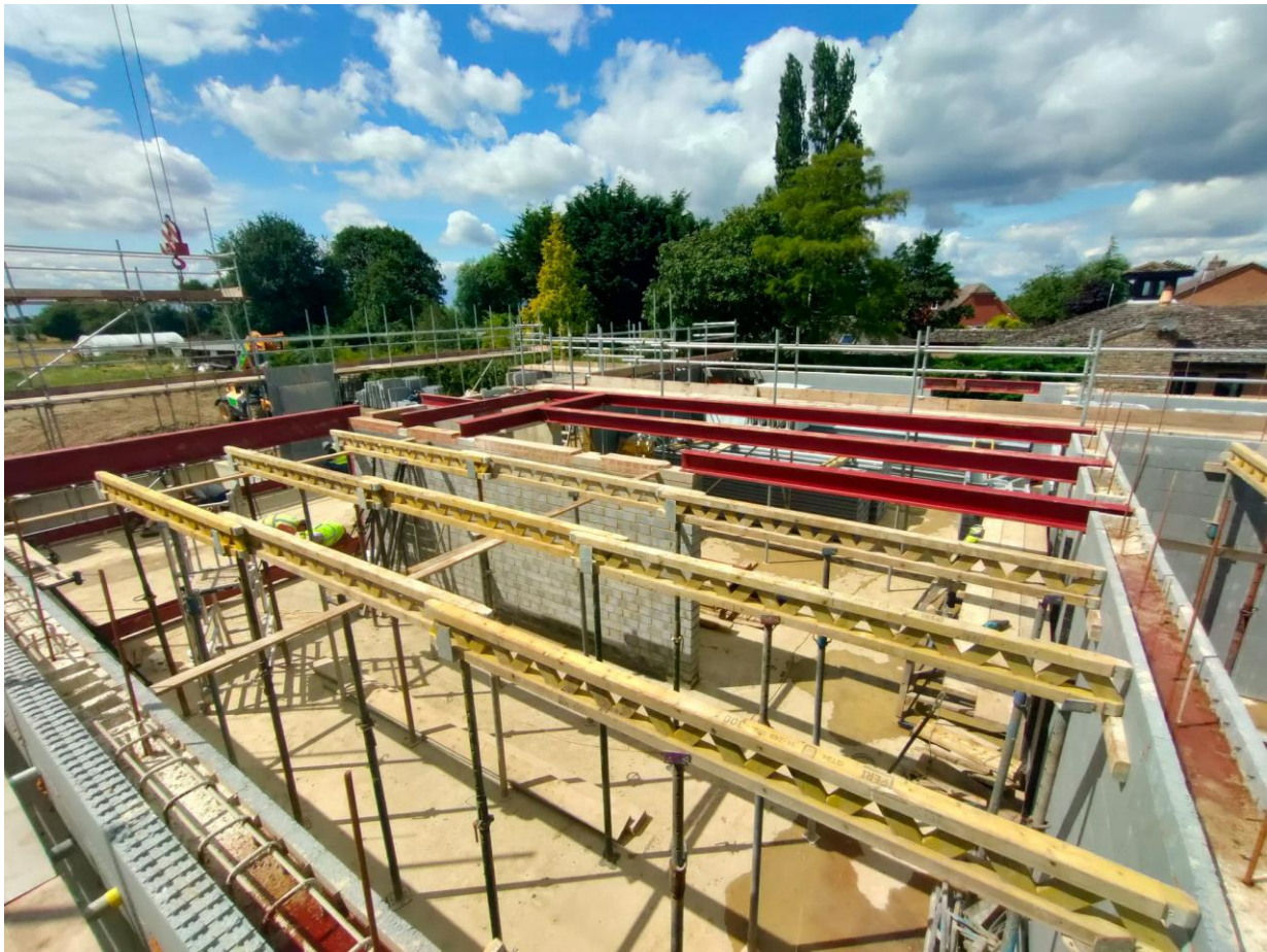
TF7 - Typical Thermofloor Propping Support prepared to take floor above
