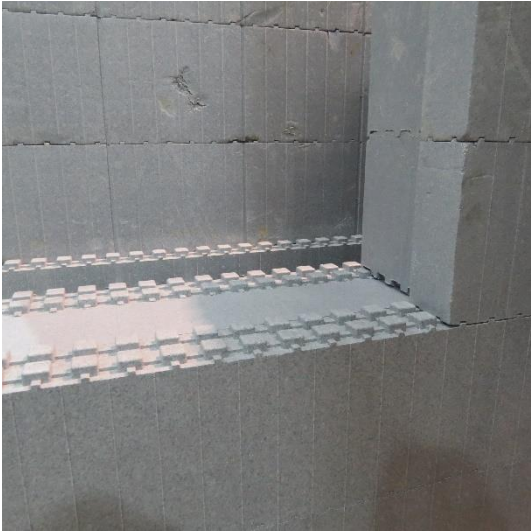
Window opening before preparation
