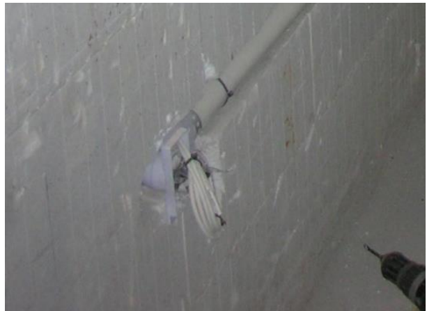
Installation of Large Conduit
