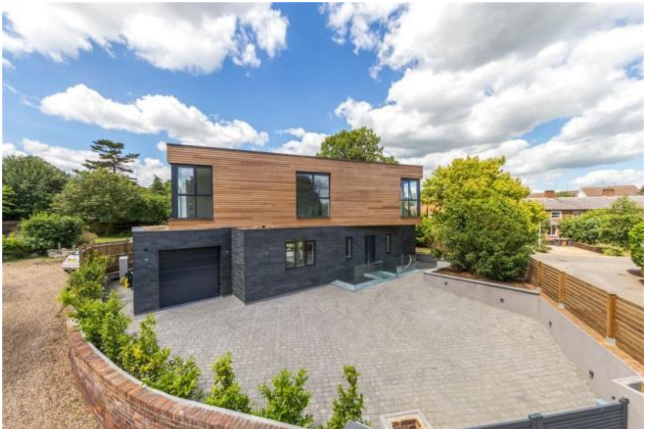
Timber Cladding with Stone Tiled walls
