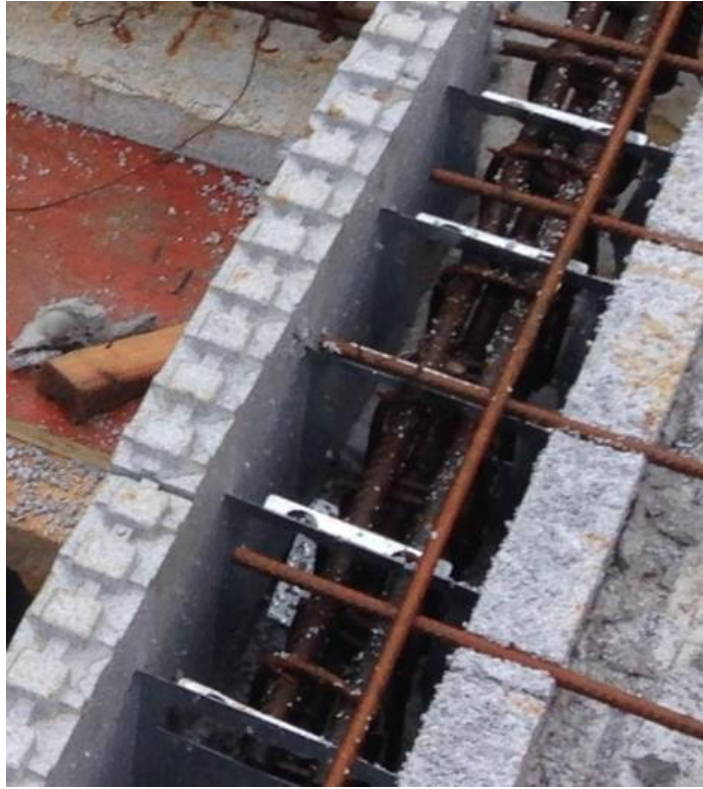
Lintel Steel Reinforcement (incorporating flooring mesh)
