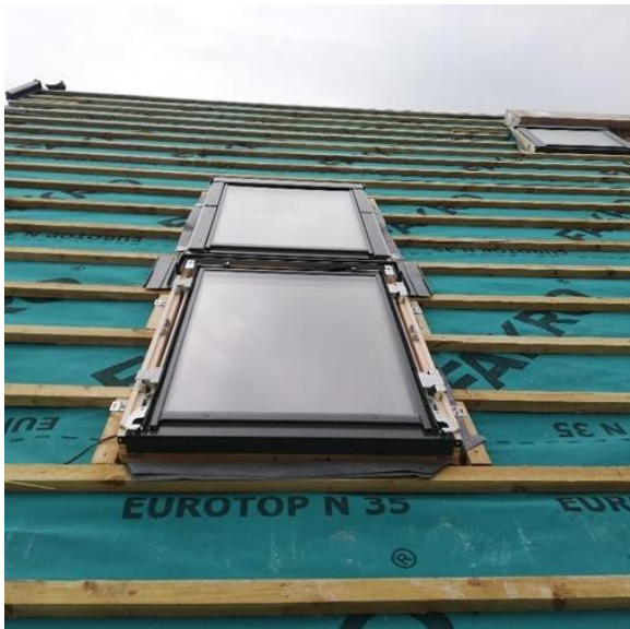
Typical window framing in ThermoRoof Panels
