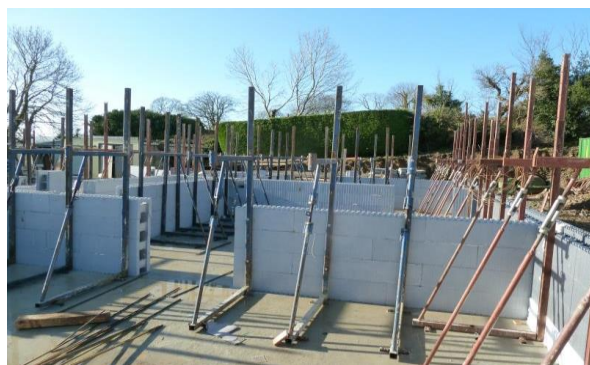
Fig 11. Wall alignment props
