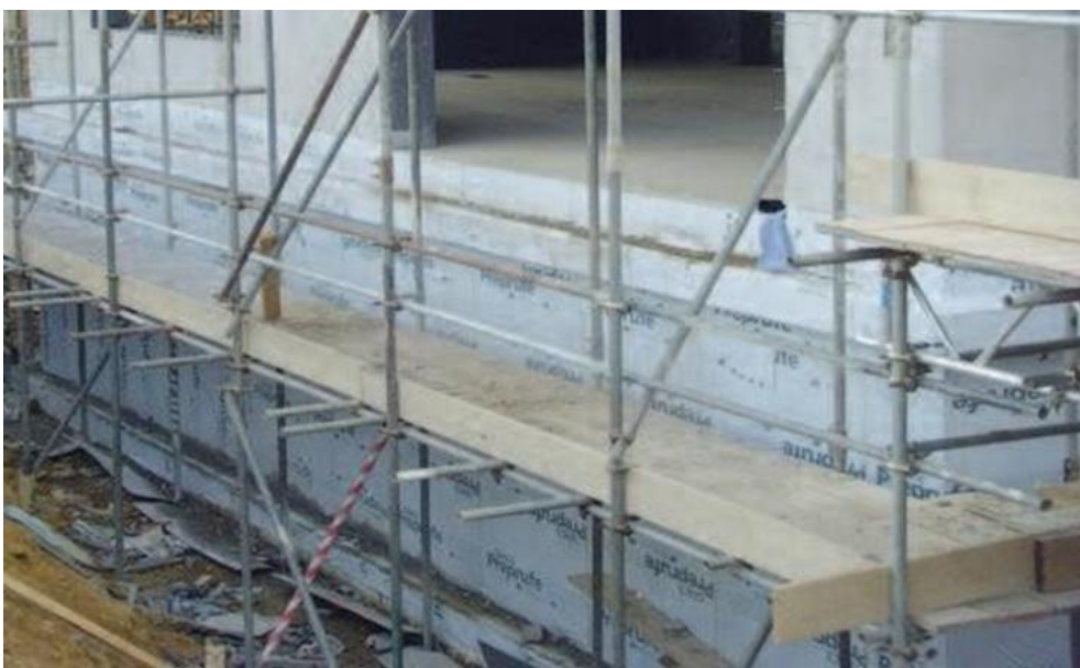
Typical Tanking membrane detail
