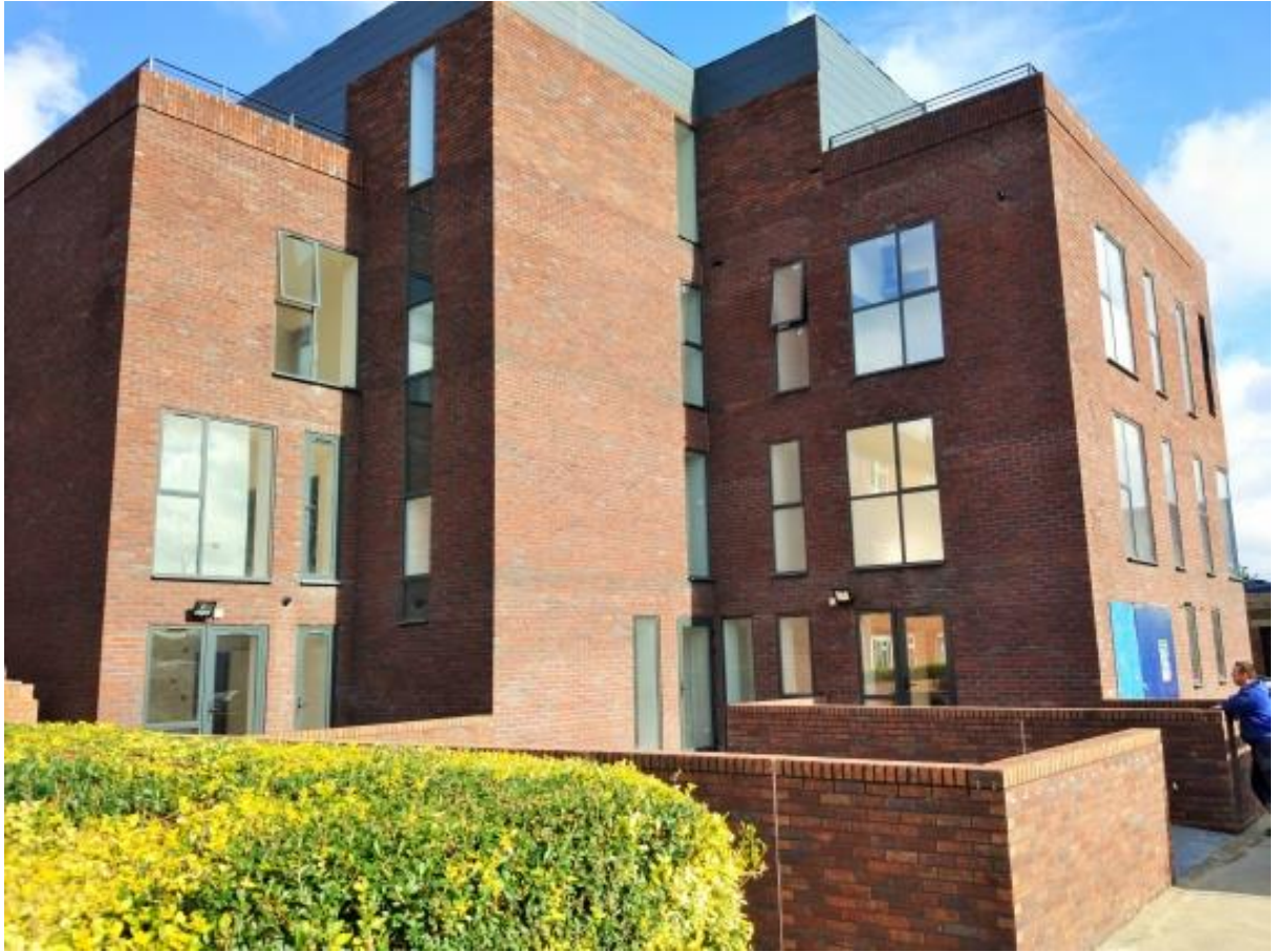
Full Brick Finish to Apartment block
