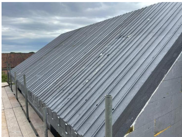
Straight A-Line roof running gable to gable
