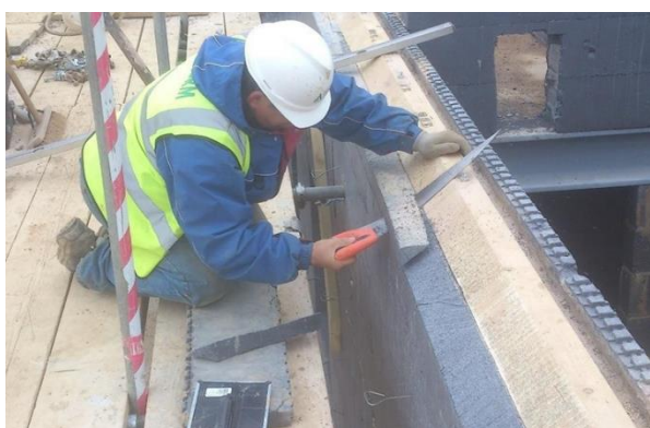
EPS Chamfer for Seal To ThermoRoof Panel
