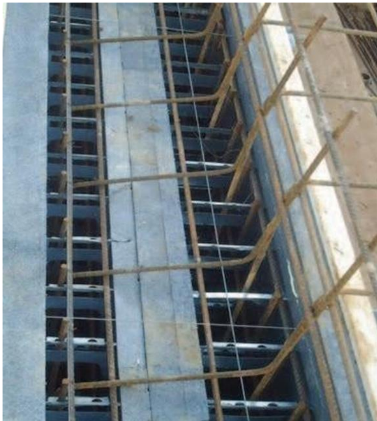
First Storey Basement Wall (650mm Double Wall) The second storey was erected with a single basement 350mm
