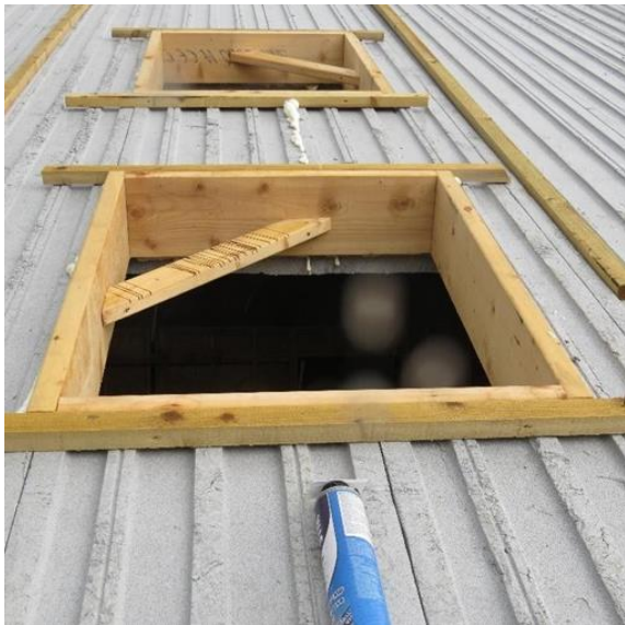
Typical window framing in ThermoRoof Panels
