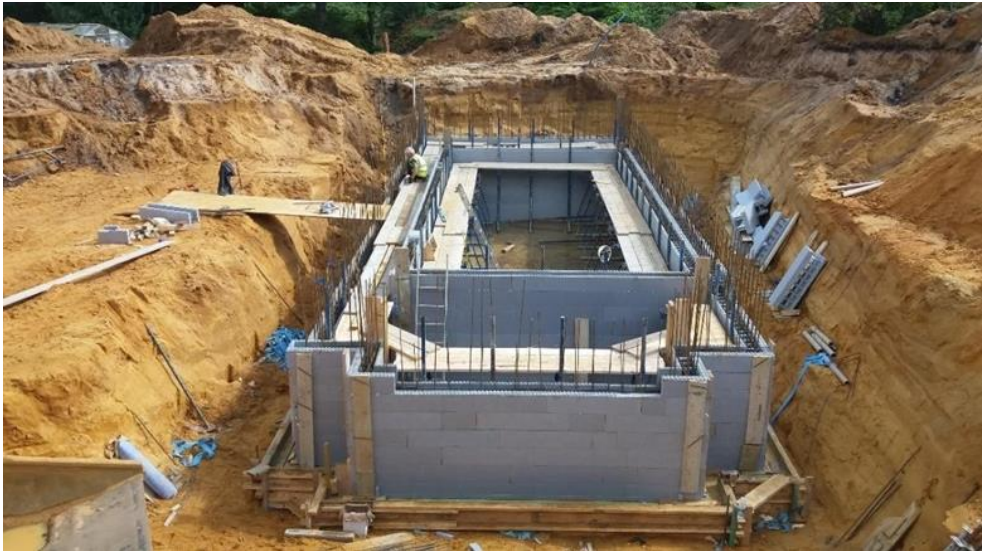
Lower Basement Incorporating Swimming Pool
