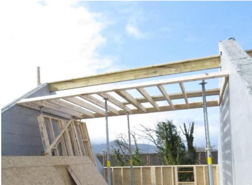
Pre-Fabricated Collar Ladder Positioned before panel placement
